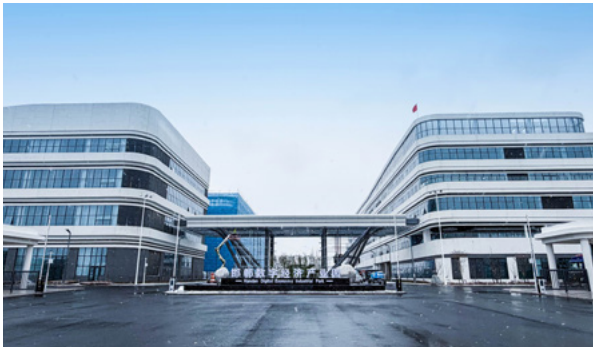
河北邯郸数字经济产业园 Handan Digital Economy Industrial Park, Hebei
